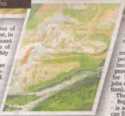
Aerial views of on-going work at Bujagali Hydro-power Project. COURTESY PHOTOS.
